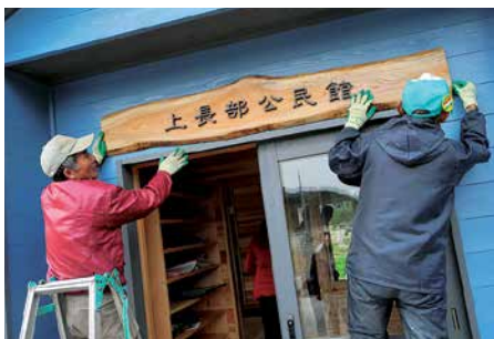
Carpenters from the village of Osabe, Rikuzentakata, install a sign for a new community center donated by Germans.
